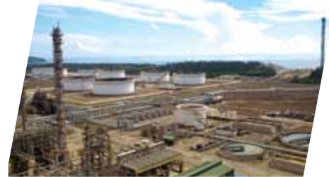
Oil-and-Gas, Chemical & Utility Plant Maintenance
